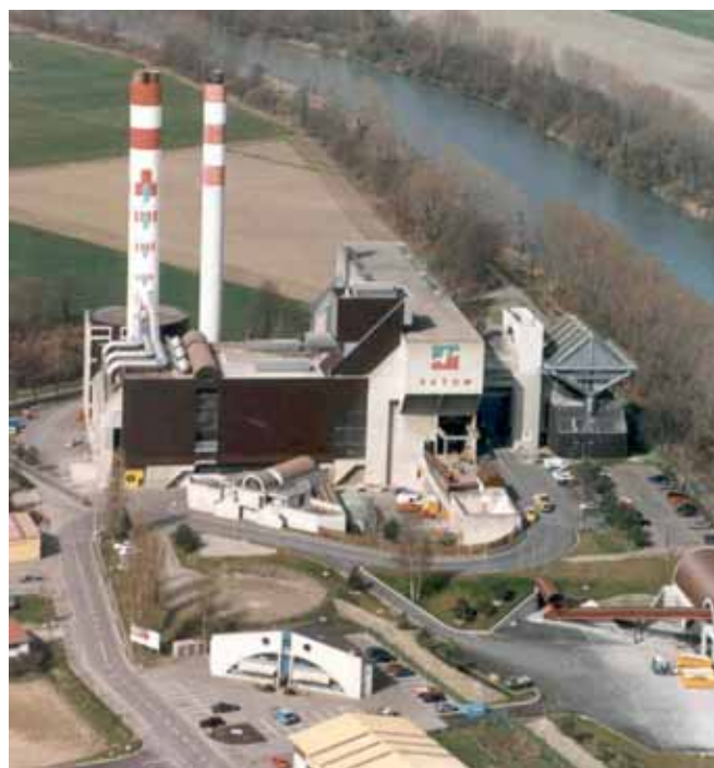
Abb. 8 KVA SATOM Monthey (CH)
